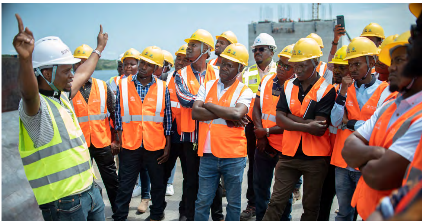
The TANROAD construction supervisor at the bridge, Eng. William Benedict Sanga gives an insight about the on going construction of Kigongo-Busisi bridge to GGML engineers during the visit.
